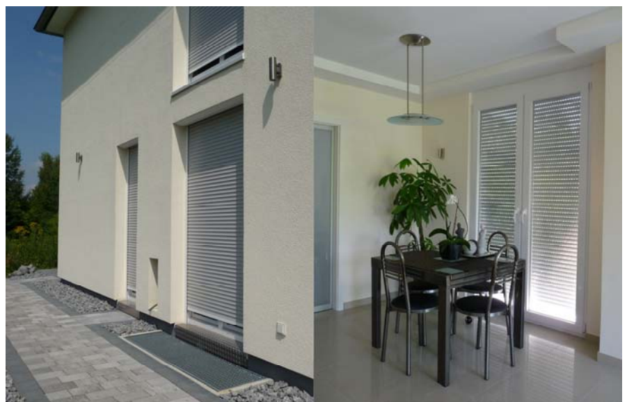
Automatic shading - outside exact positioned roller shutters, inside cool and light
